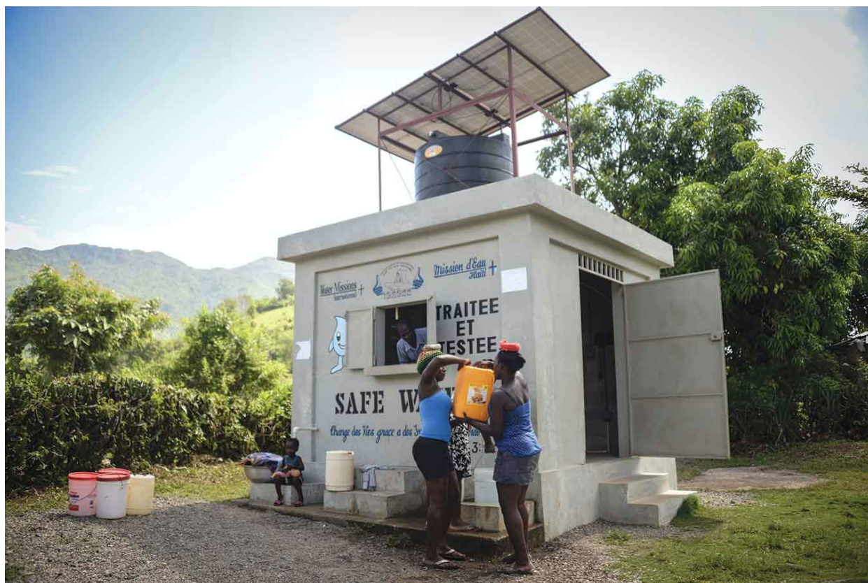
Figure 13. Solar Water Well, Treatment, and Storage
